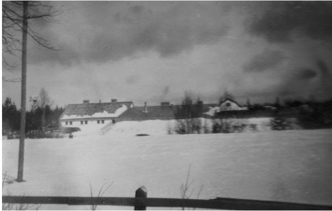
Water Purifying Plant in Vasa, Finland
